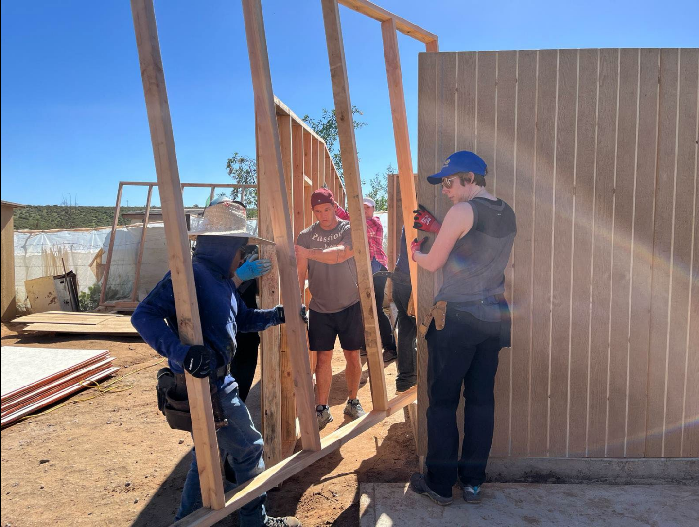
Three layers - centre wall built on top of already assembled side and end walls
