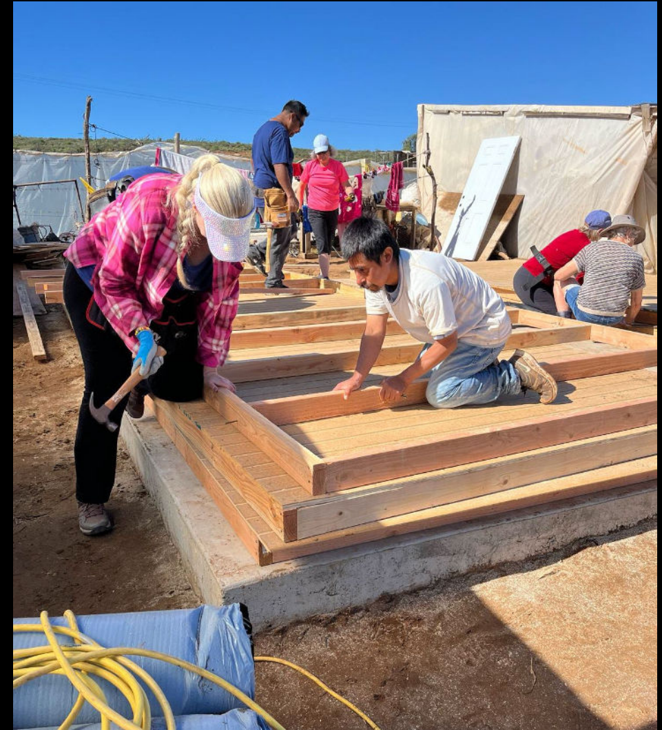
Three layers - centre wall built on top of already assembled side and end walls
